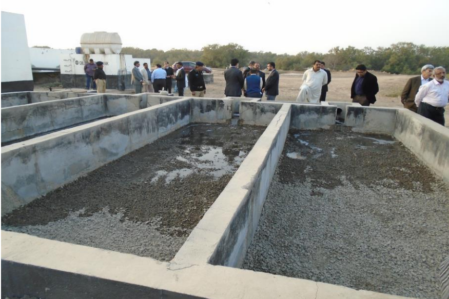
DRY SLUDGE TANKS TREATMENT PLANT AT BIN QASIM
