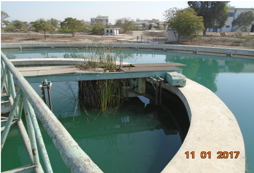
NON FUNCTIONAL CLARIFIER AT COD FILTER PLANT
