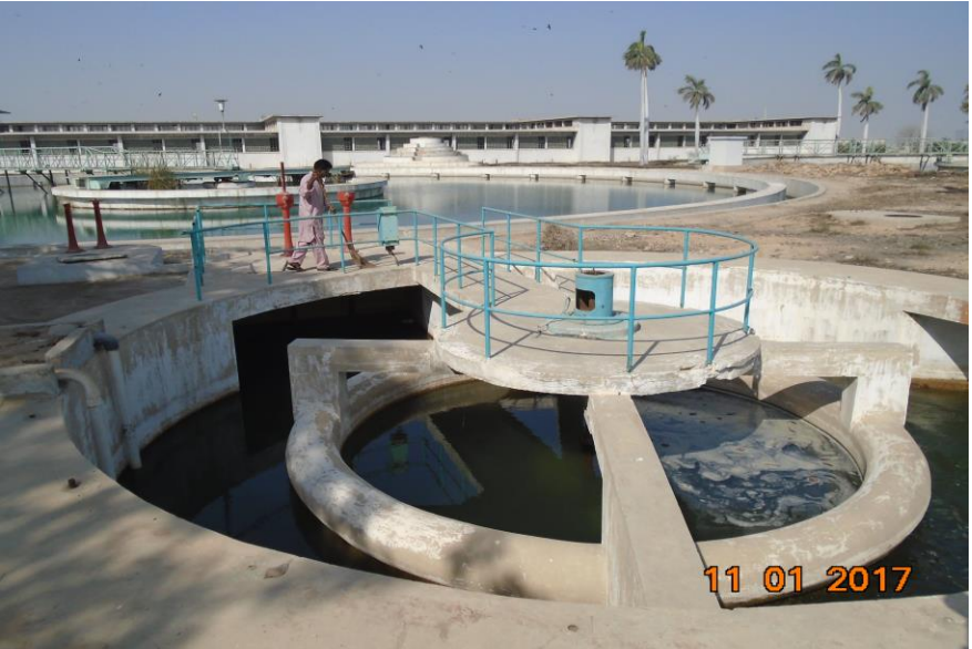
CLARIFIER AT COD FILTER PLANT
