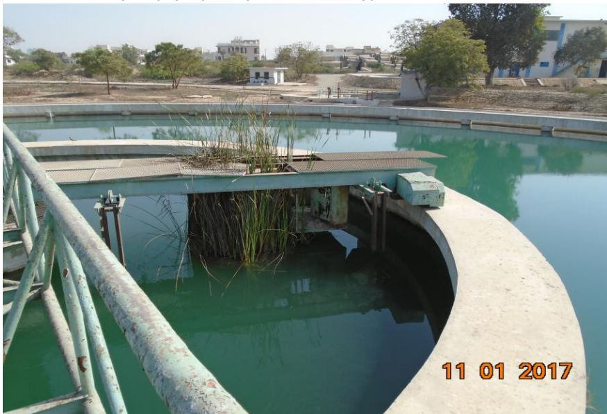
NON FUNCTIONAL CLARIFIER AT COD FILTER PLANT
