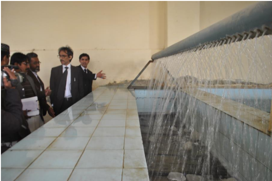
MIXTURE OF ALUM AT KOTRI FILTER PLANT
