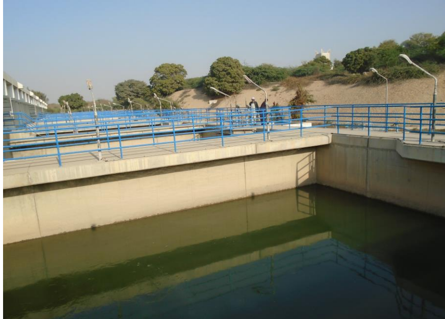
CLORINATING TANKS AT NEK FILTER PLANT
