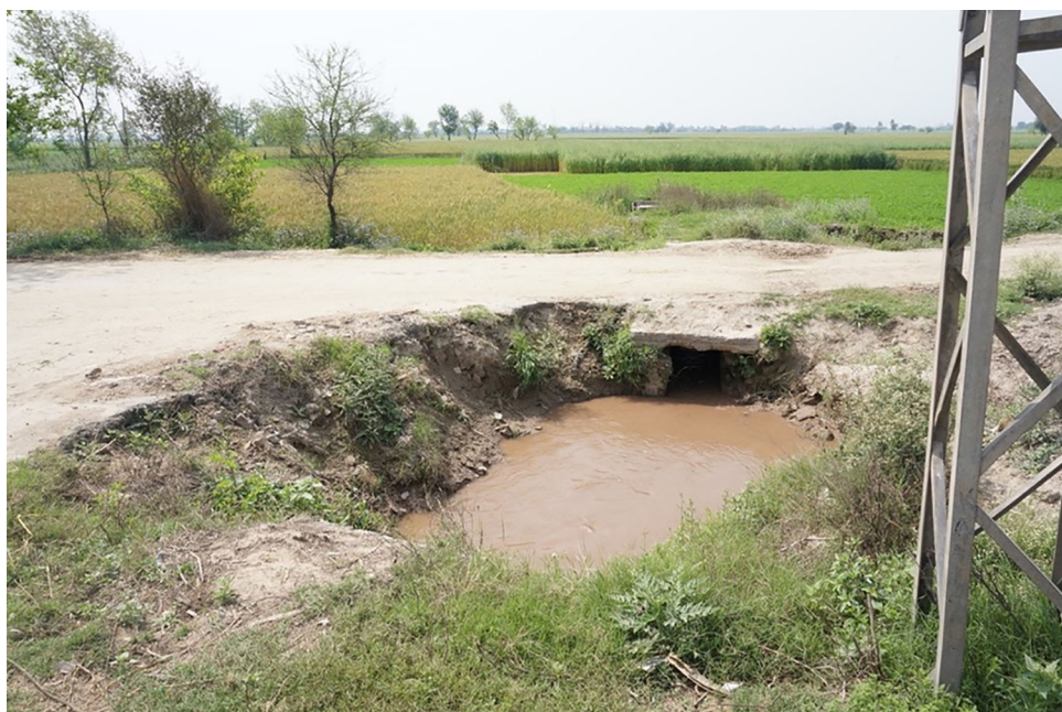
Figure 1: Moga is the name for the outlet. It is also called sluice, turnout, and offtake in some of the academic literature. The outlet is constructed to deliver the designed discharge of water from distributaries to agricultural fields through water courses. It is also the node in the infrastructure which marks the end of the Irrigation Department's property and jurisdiction. (source: photograph by author)
