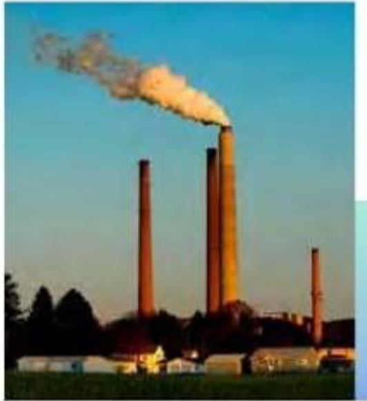
The A.E.P. (American Electric Power) coal burning plant in Conesville, Ohio. Michael S. Williamson/The Washington Post
