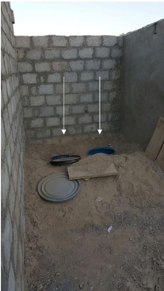
Blue Drums Buried in the Ground
