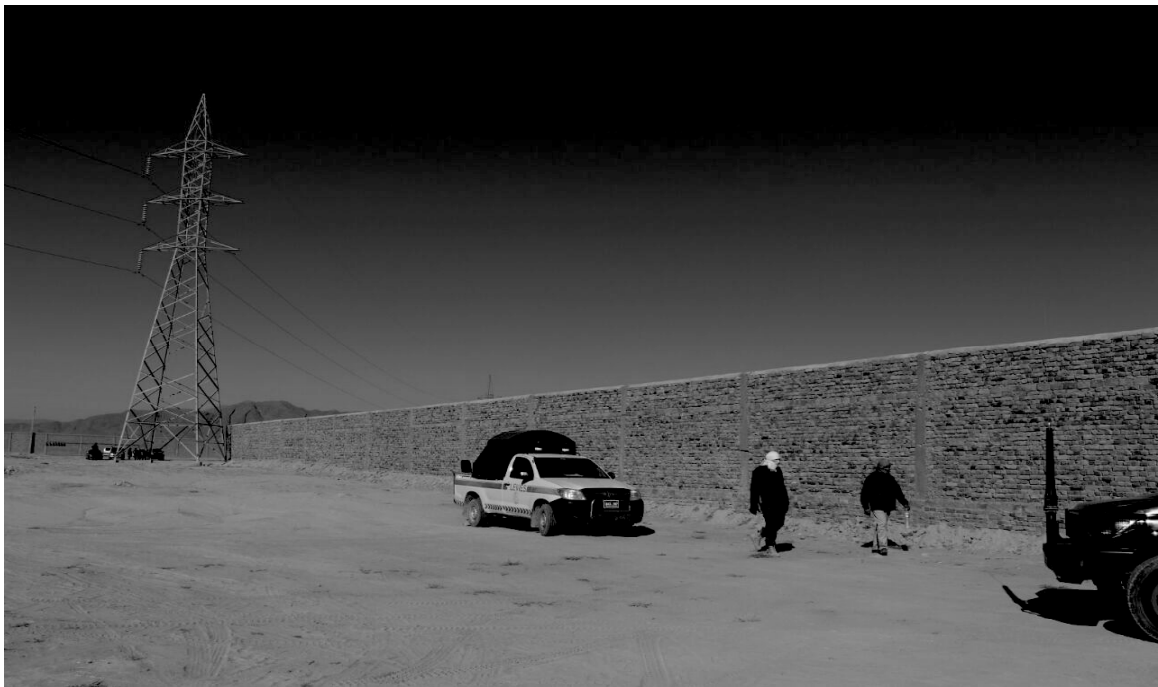
Side view of wall
